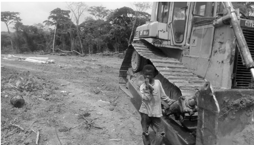
As the bulldozers cleared a swathe through the forest ...
