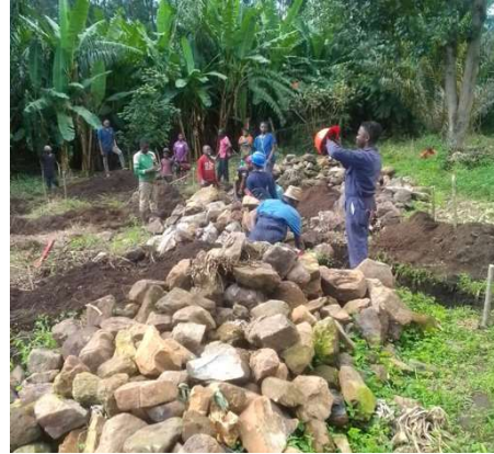
Nyarubungu School: Every construction project begins with the laying of the foundations © Claude Sikubwabo
