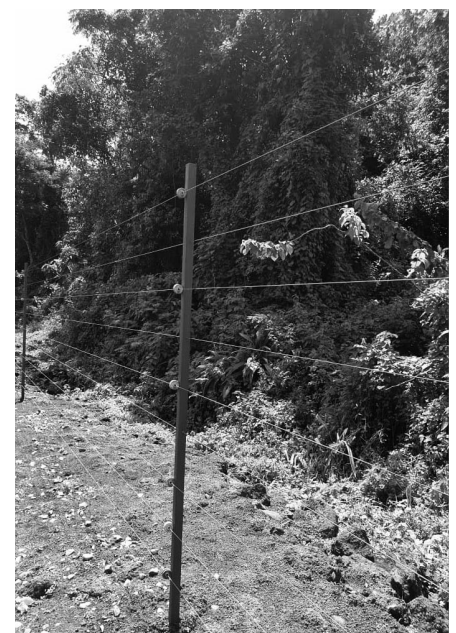
Close-up of the electric fence
