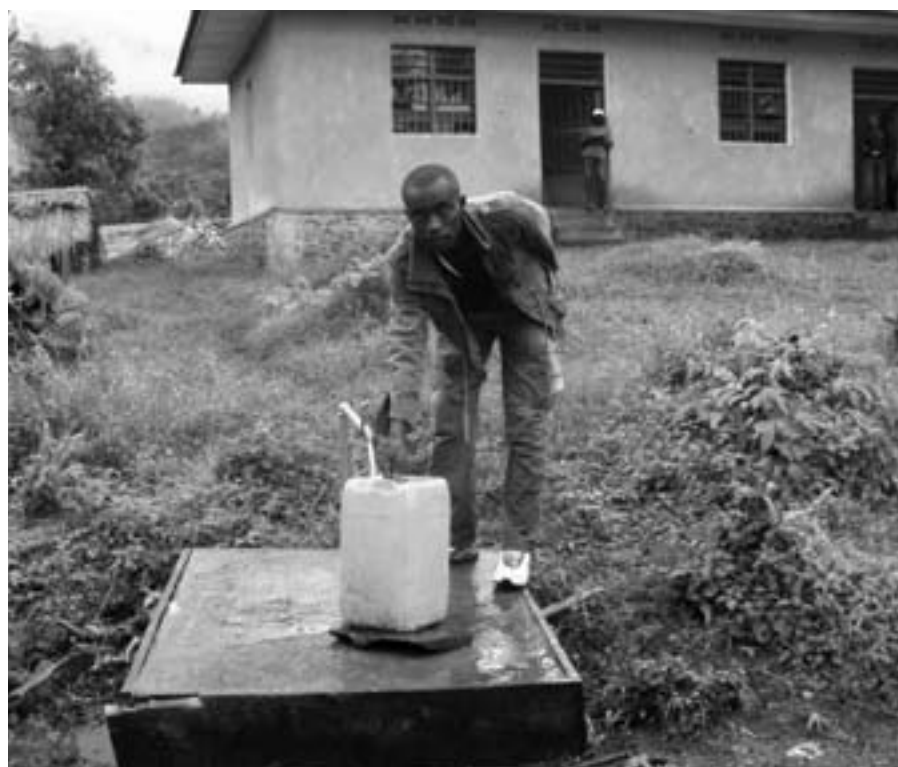
The water for the Sarambwe patrol post is flowing!
