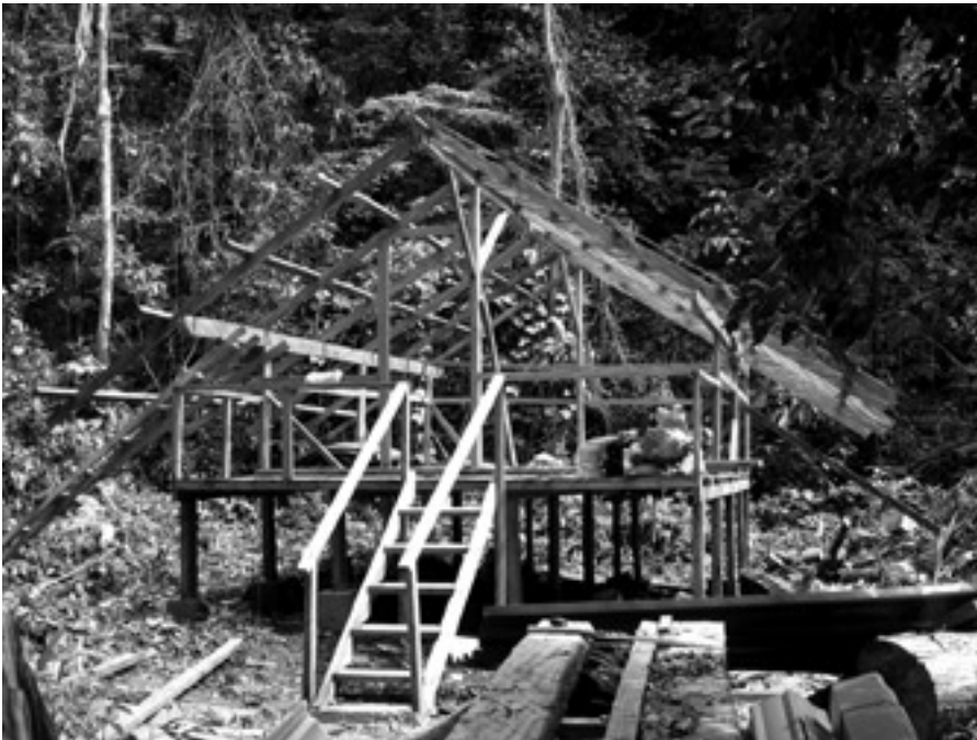
The new camp in Mbe is constructed
