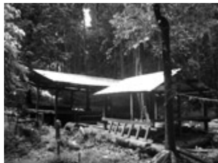
New buildings at the Afi ranger camp
