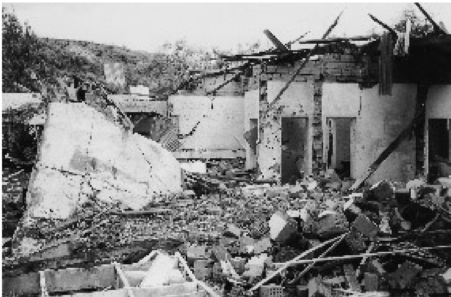
The building of the WWF education program for the Virunga National Park in Goma after a bombing raid in May 1999
